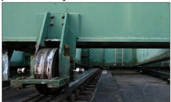
Below: The wooden longitudinal sleepers have been exchanged for metal replacements, on which the rails will sit.
